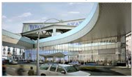
STV Incorporated Left, a rendering of the renovated George Washington Bridge Bus Station, which is to be completed by spring 2013.
