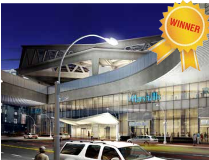
Photo: Courtesy of Port Authority of New York and New Jersey/SJM Partners, Inc. A $183 million redevelopment effort by the Port Authority of New York and New Jersey to revitalize the George Washington Bridge (GWB) Bus Station, a transportation hub in New York City.
